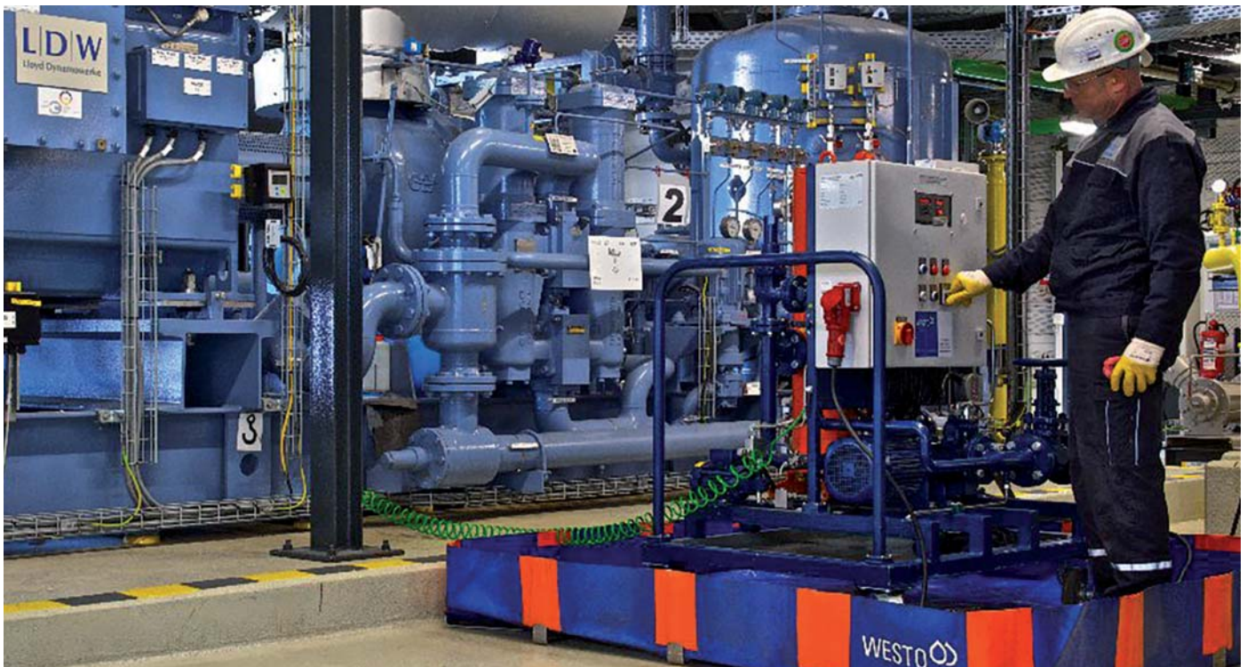
Jointly developed by WESTO and Currenta: a partial flow filter system specially designed for the screw compressors used in refrigeration that takes into account the proportion of ammonia (NH 3 ) in the oil circuit.
