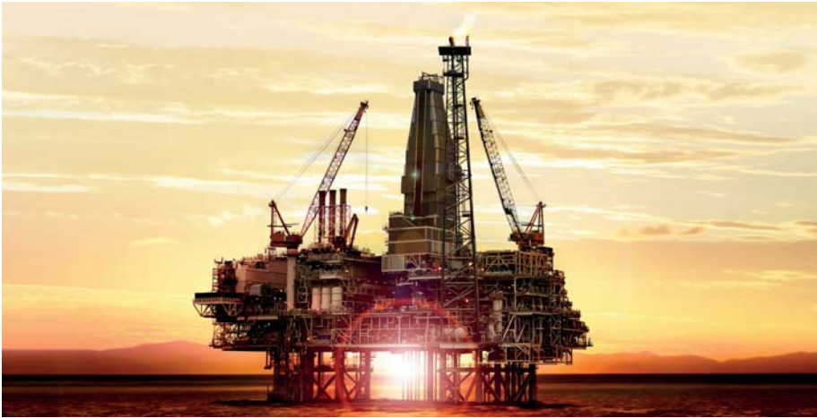
Drilling rig in the South Chinese Sea. The power is supplied by a 26 MW gas turbine.
